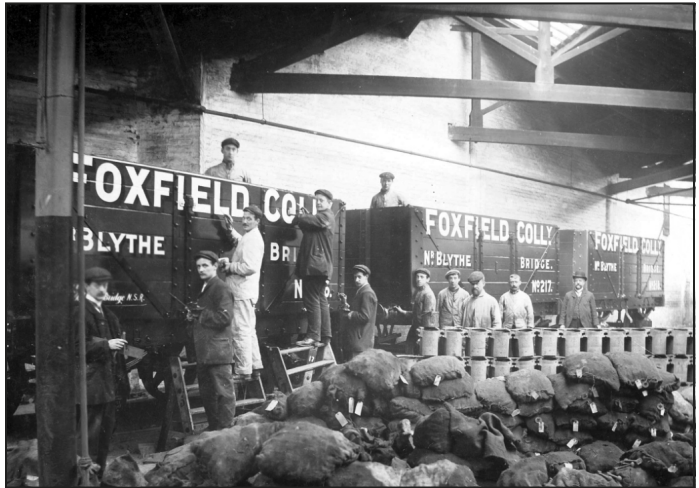
Above Early production at the L&Y wagon works Heywood. Sign writing on a build of coal wagons for the Foxfield Colliery Staffordshire during 1906. Photo Reddy family collection.
